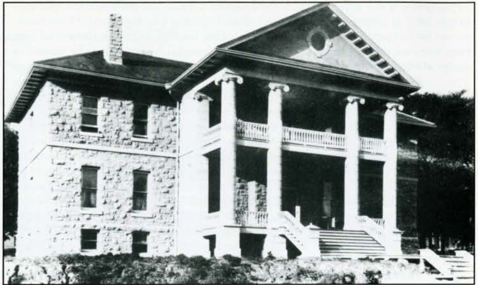
Figure 8. Front elevation of the nurses' home, Kingston General Hospital, soon after its completion in 1904. (Queen's University Archives)
