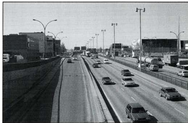
Figure 1. Metropolitan Boulevard, Montreal, begun 1958-60. (Y. Deschamps, 1997)
