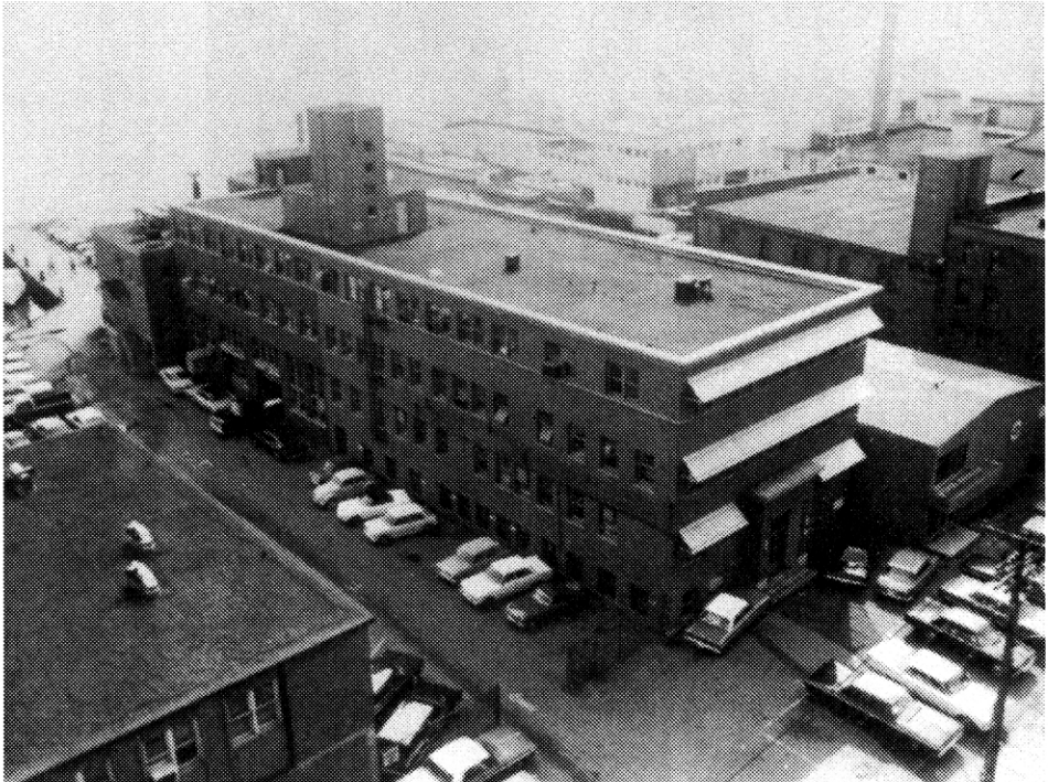
Fig 2. The much modified final form of the building at 1707 Lower Water Street in the 1970s (by then known as the Halifax Fisheries Research Board Laboratory). At its peak in the 1960s it provided facilities for around 90 staff.
