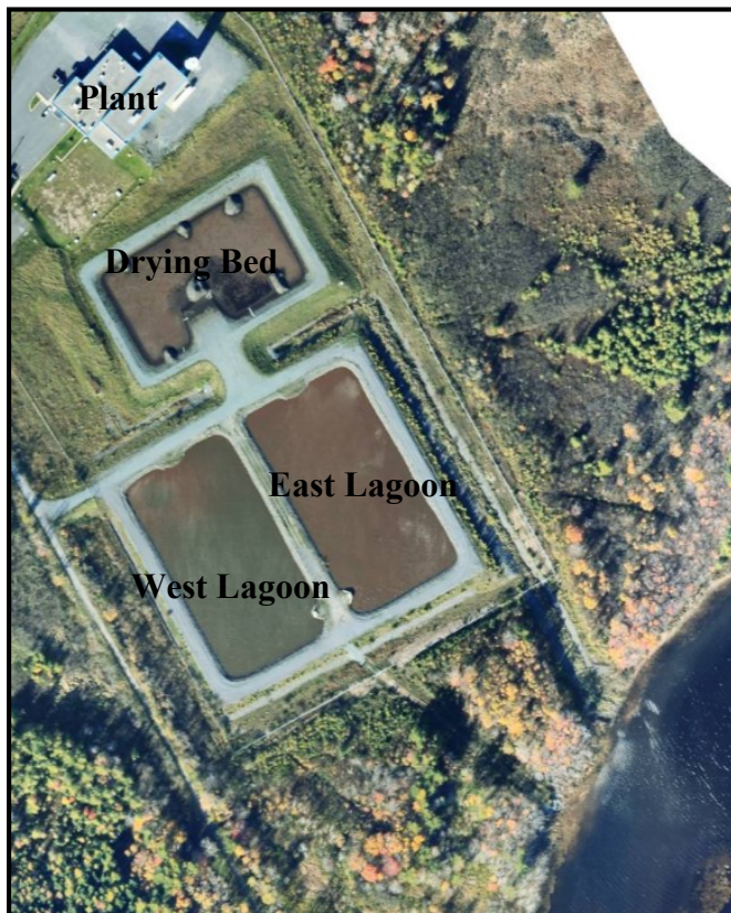
Figure 7 Orthophotograph of the WTP, Lagoons and Drying Bed
