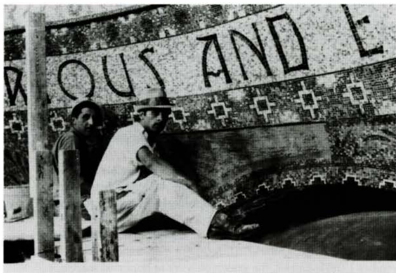
Fig. 1. Two workers (Remo De Carli on the right) install the mosaics below the dome of the Foster Memorial in Uxbridge, Ontario, in 1936. (Private collection)
