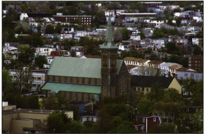
Fig. 4. St. John's, Newfoundland, St. Patrick, exterior NW (SW). (Photo: Malcolm Thurby)
