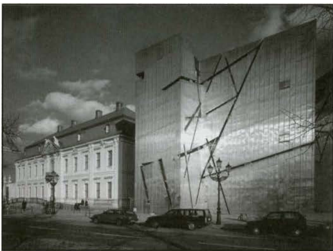
Fig. 6. Liebeskind, facade, Jewish Museum, under construction (1997). (James Young, At Memory's Edge )
