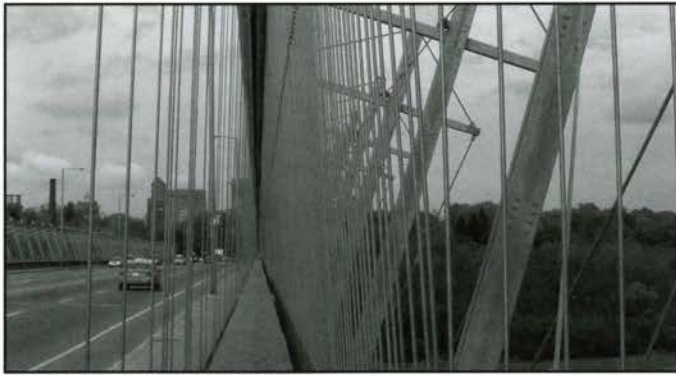
Fig. 8: View between layers of steel cable. (Photo: Marco Polo)
