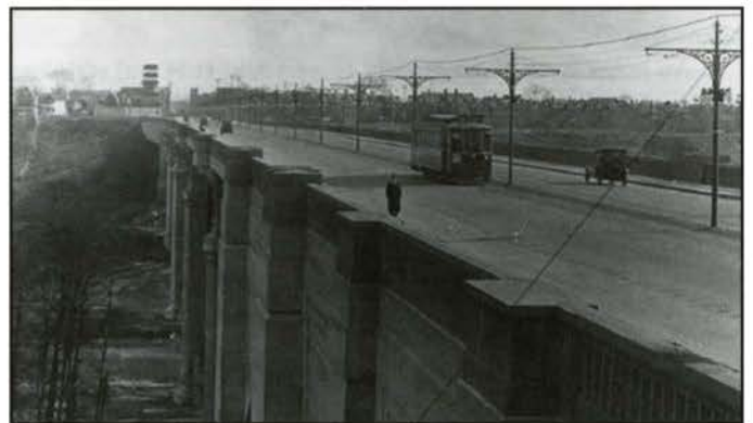
Fig. 15: The original baluster and handrail were very modestly scaled in relation to the grand viaduct. (City of Toronto Archives)
