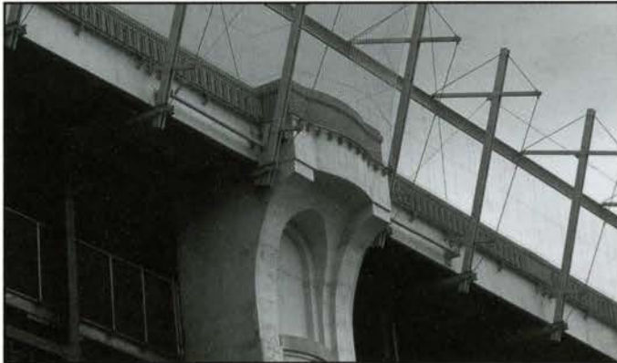
Fig. 9: Typical lookout at top of bridge pier. (Photo: Marco Polo)
