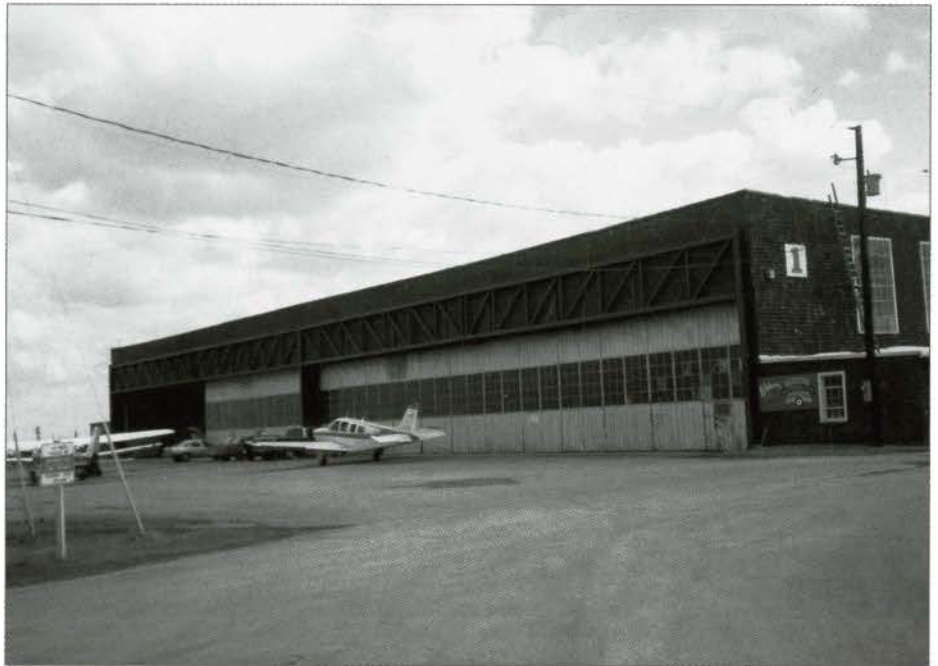
FIG. 8. BRANDON, MANITOBA. HANGAR NO. 1, NORTH ELEVATION | STEPHEN HAYTER, 1999
