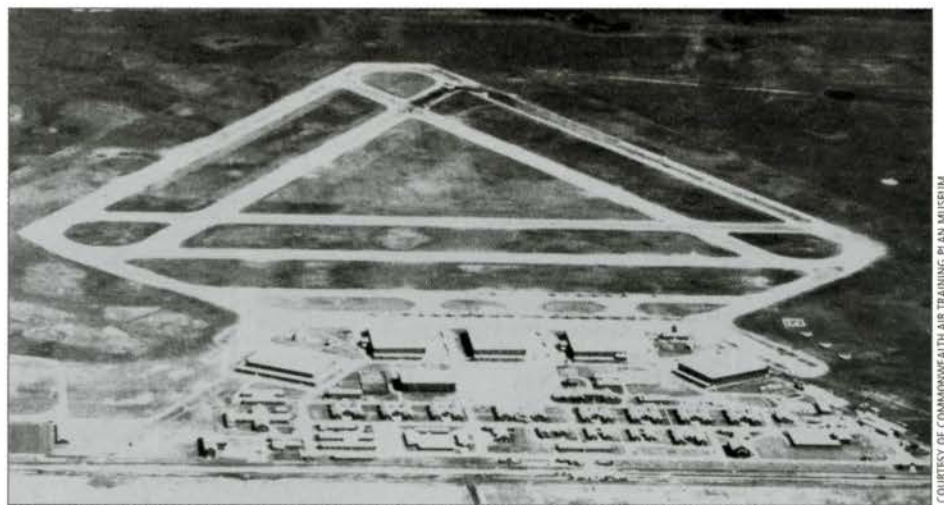
FIG. 7. BRANDON, MANITOBA. AERIAL VIEW, SFTS 12, CA. 1941-45. HANGAR NO. 1 IS ON THE EXTREME LEFT.
