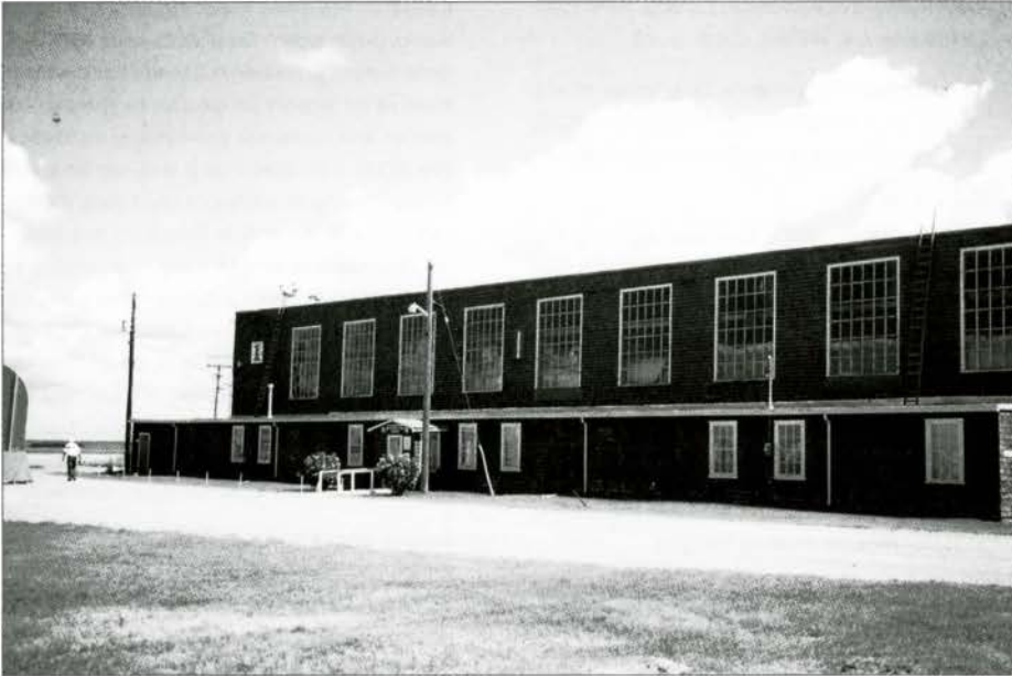
FIG. 12. BRANDON, MANITOBA. HANGAR NO. 1, WEST (FRONT) ELEVATION | STEPHEN HAYTER, 1999
