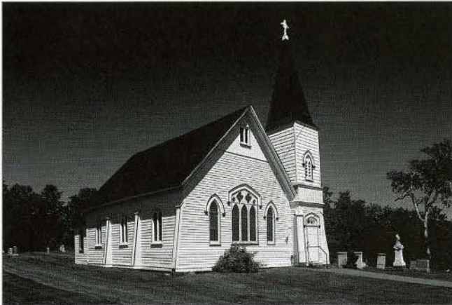
FIG. 49. SPRINGFIELD, ST. ELIZABETH. EXTERIOR FROM NW (SW). | Malcolm Thurlby.
