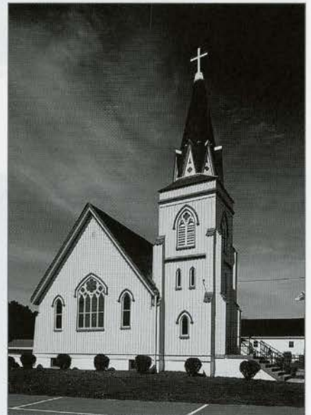
FIG. 48. KENSINGTON, ST. MARK, 1885. W FAÇADE. | Malcolm Thurlby.
