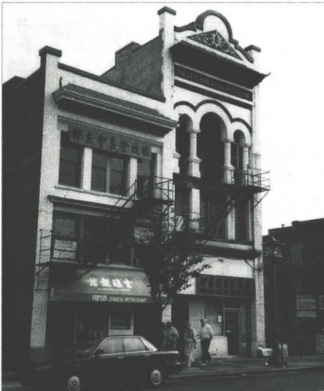
FIG. 27. THE SHON YEE AND LEE BENEVOLENT ASSOCIATION BUILDINGS IN VICTORIA. | EDWARD MILLS, PARKS CANADA, 1995.
