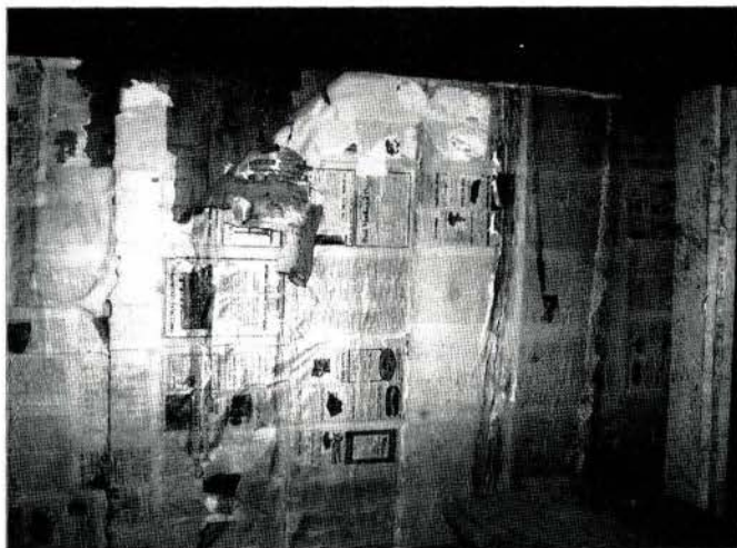
FIG. 23. AN EXAMPLE OF WALL COVERINGS FROM THE BARKERVILLE CHEE KUNG TONG BUILDING. | NORMAN SHIELDS, PARKS CANADA, 2006.
