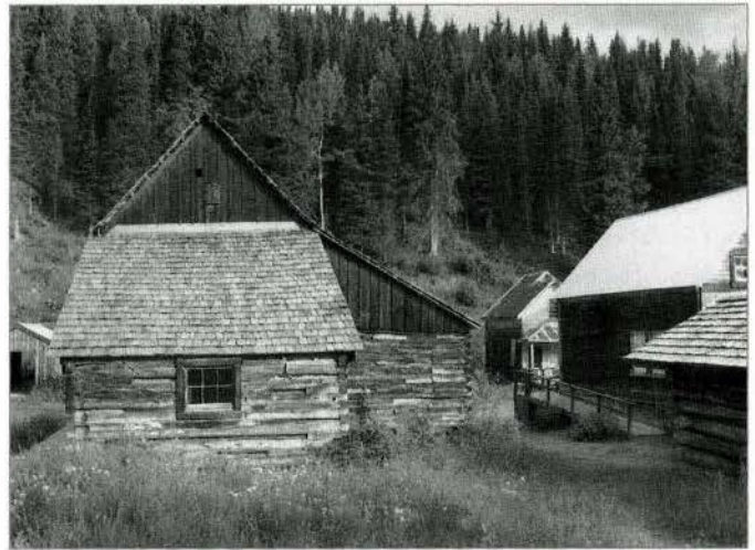
FIG. 3. THE EAST LEAN-TO ADDITION (BUILDING 84C) WAS ERECTED CA. 1883 AND SERVED PRIMARILY AS A KITCHEN. | NORMAN SHIELDS, PARKS CANADA, 2006.
