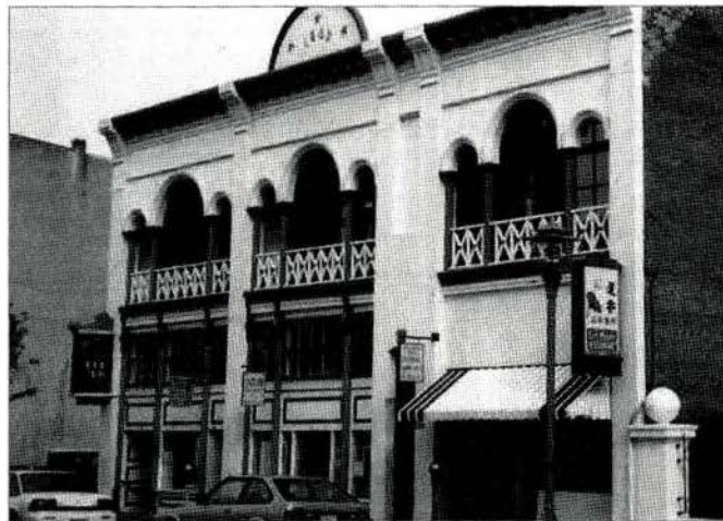
FIG. 26. THE GEE TUCK TONG BENEVOLENT ASSOCIATION BUILDING IN VICTORIA. | EDWARD MILLS, PARKS CANADA, 1995.
