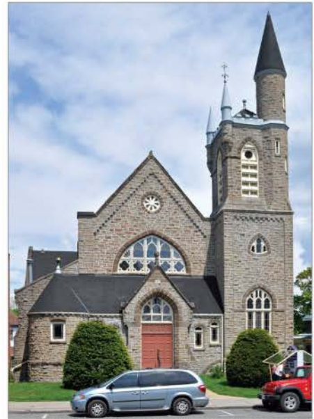
FIG. 18. ST. ANDREW’S PRESBYTERIAN CHURCH, CARLETON PLACE, ONTARIO, ARCHITECT SIDNEY BADGLEY, 1886. | JENNIFER MCKENDRY, 2012.
