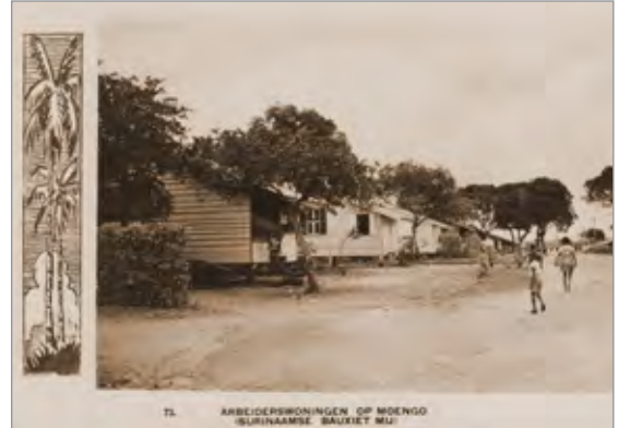
FIG. 48. POSTCARD OF THE WORKERS' HOMES IN MOENGO, AGAIN IN THE "TROPICAL BUNGALOW" FIGURE, HOWEVER, ERECTED ON STILTS HERE; THIS IS ALSO THE CASE, AT THE SAME TIME AND NO DOUBT FOLLOWING THE RECOMMENDATION OF MORRIS KNOWLES, IN MACKENZIE. | PRIVATE COLLECTION.
