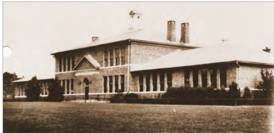
FIG. 43. THE NEGRO SCHOOL BUILDING COMPLETED IN 1925, LISTED IN BADIN'S PROPERTY FILE. THE NOTICE INDICATES THAT GRAMMAR AND HIGH SCHOOL SUBJECTS ARE TAUGHT, AND THAT THE ROOF, GUTTER AND DOWNSPOUTS ARE ENTIRELY MADE OF ALUMINUM. | BHM.
