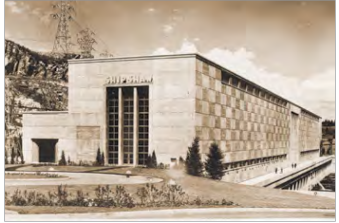
FIG. 19. THE SHIPSHAW II HYDROELECTRIC POWER PLANT, BUILT ACCORDING TO JAMES CURZEY MEADOWCROFT'S PLANS IN 1942, WHICH CAN BE SEEN ON ONE OF THE MANY POSTCARDS BEARING ITS IMAGE. | BANQ (QUEBEC).
