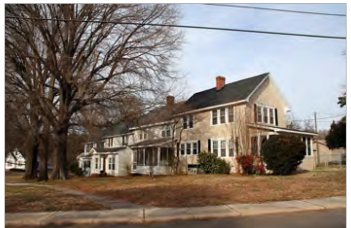
FIG. 6. A FOUR-UNIT DWELLING OF BADIN; NOTE THE UNBOUNDED LOT. | LUCIE K. MORISSET.
