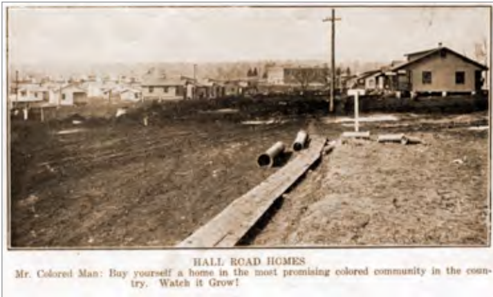
FIG. 34. ADVERTISEMENT FOR HOUSES AIMED AT "MR. COLORED MAN" IN ALCOA, TENNESSEE. | BCHGS.
