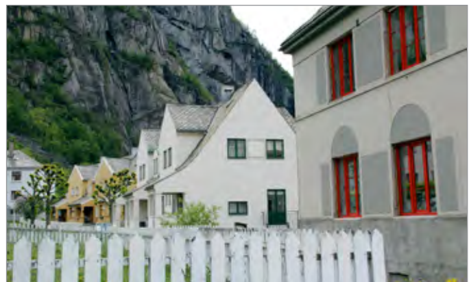
FIG. 61. HOUSES IN THE TVEITAHaugEN NEIGHBOURHOOD, IN THE ALUMINUM CITY OF TYSSedal, CONSIDERED AS ONE OF THE FIRST NORWEGIAN GARDEN CITIES; THEY WERE BUILT ACCORDING TO THE PLANS OF ARCHITECT OSCAR HOFF BASED ON A GENERAL PLAN BY MORGENSTIERNE & EIDE. | LUCIE K. MORISSET.
