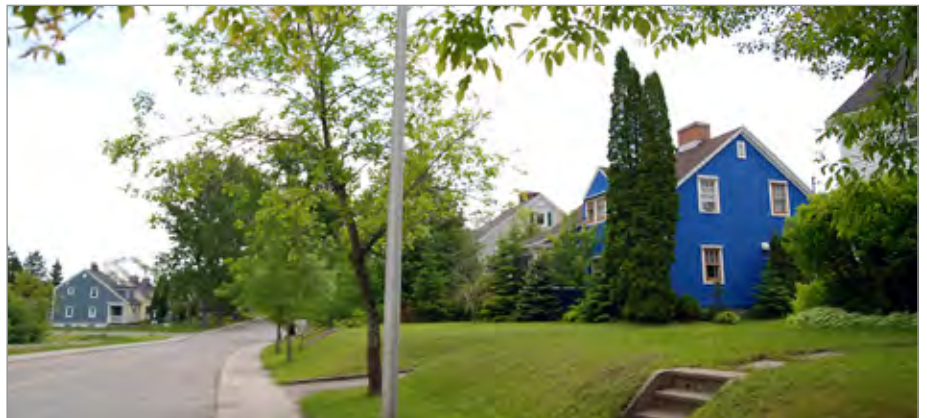
FIG. 64. VIEW OF PART OF RUE RADIN (WHICH BECAME LA TRAVERSE), WHOSE ROUTE FOLLOWS AN OLDER COUNTRY ROAD AND WHOSE LOTS REMAINED UNREGISTERED UNTIL THE END OF THE 1930S: THE TWENTY-SOME HOUSES WHICH CONSTITUTE THE COMPANY'S "PRIVATE DOMAIN." | MARIANNE CHARLAND.
