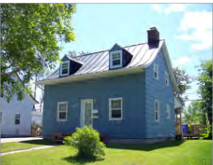
FIG. 51. A HOUSE OF THE A1 MODEL OF ARVIDA, RECOGNIZABLE BY ITS ROOF EAVES AND ITS GABLED DORMER WINDOWS. | JOANIE LAPOINTE.
