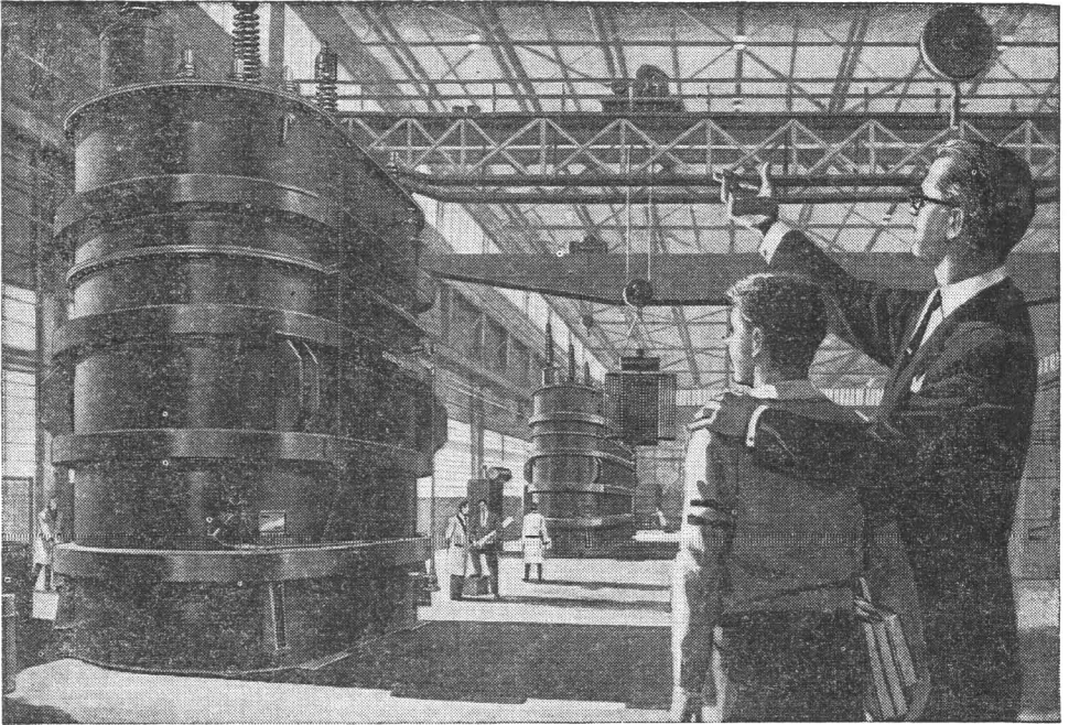
A scene in the Company's new Works at Guelph, Ontario... the largest power transformer plant in Canada. Here, transformers are built for the country's great electric power projects. Many thousands of mathematical calculations are involved in designing transformers, and the wide variety of other electrical equipment manufactured at Canadian General Electric's fifteen plants.
