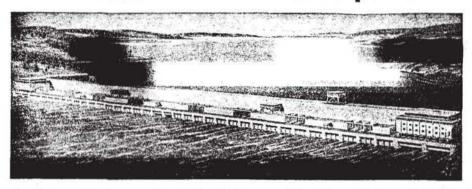
Artist's conception of the St. Lawrence River Power Project. One of the world's greatest hydro-electric sources, it will develop 2,200,000 horsepower shared equally between Canada and the United States. The powerhouse dam will be about three-quarters of a mile long. 24 of the 32 generators will bear the famous G-E monogram—16 in the U.S. section and S on the Canadian.
