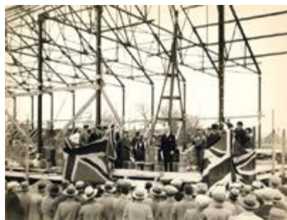
Studley Gymnasium - Hector McInnes laying cornerstone, November 1931
