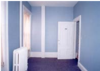
1340 Barrington Street - Hart House - Interior - Hall & Doorway, n.d.
