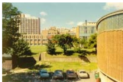
H.R. Theakston Building, October 1969
