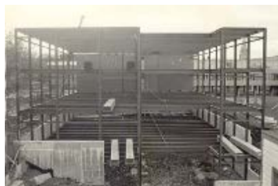
H.R. Theakston Building - Mechanical Engineering (under construction), n.d.
