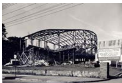
F. H. Sexton Memorial Gymnasium - Exterior - Under Construction, August 1962
