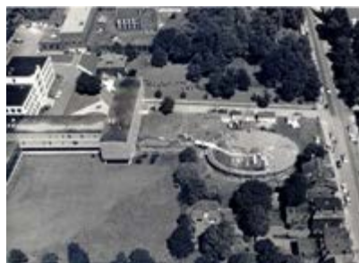
F. H. Sexton Memorial Gymnasium - Under Construction - Aerial, August 1962
