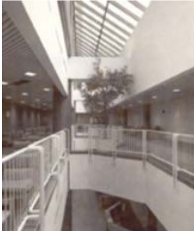
Dentistry Building - Interior - Upper Floor [2], c1980s
