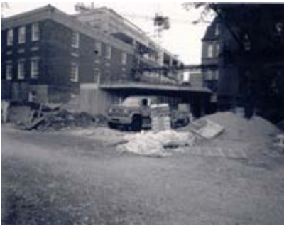
Dentistry Building Extension - Construction, October 9, 1979
