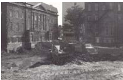
Dentistry construction begins, n.d.
