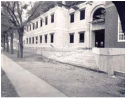
Dental Building (under construction), n.d.
