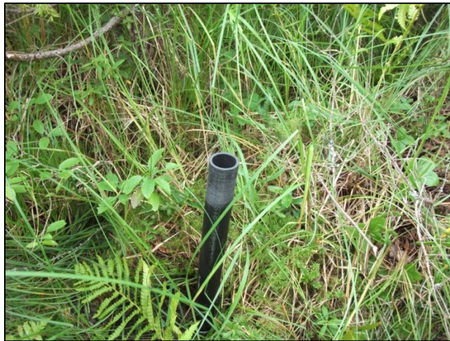
Figure 9. Shallow well installation in organic layer
