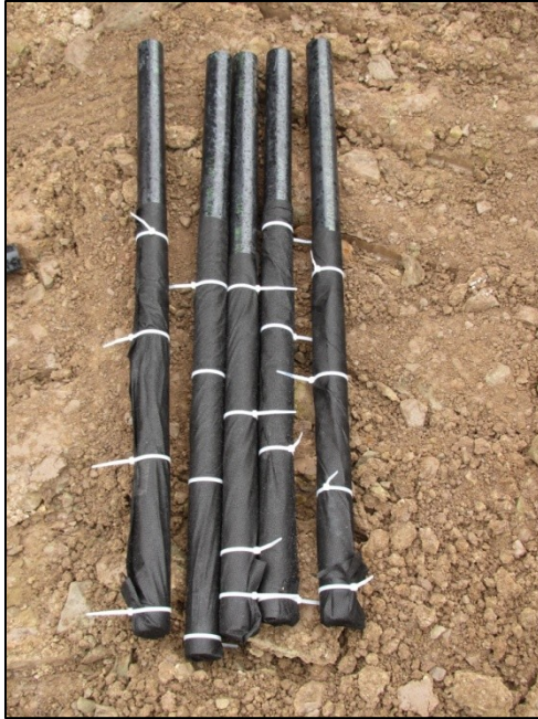
Figure 8. Constructed shallow wells
