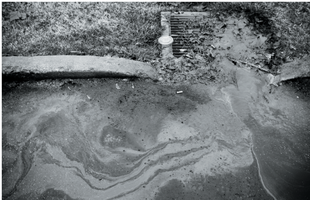
Unfiltered oil and garbage running into storm drain.
