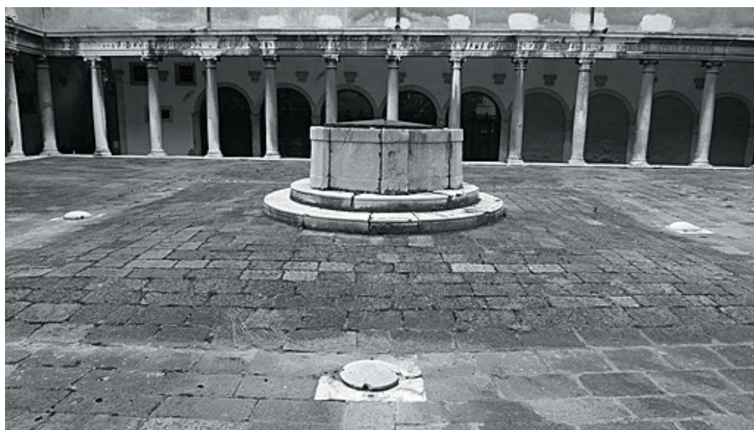
A Venetian pozzo and three visible drains; from Pries, “Drip | Dry: Systems that Seep.”
