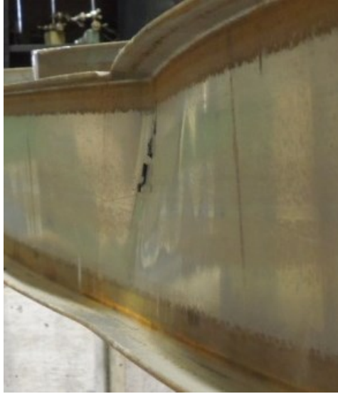
Figure 4.13 Local buckling of specimen C2 compression flange and web.
