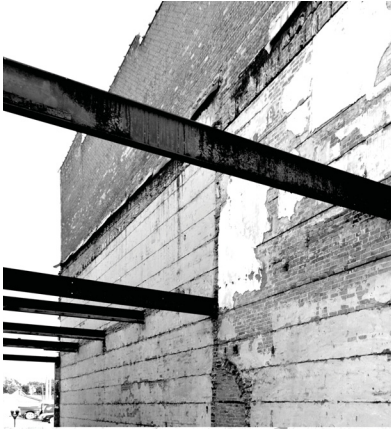
Photo of existing beams on site
