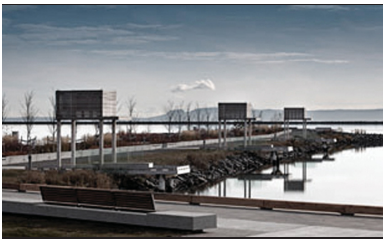
View of Pier 2, Prince Arthur's Landing, photograph likely by Brook McIlroy (Bustler 2012)
