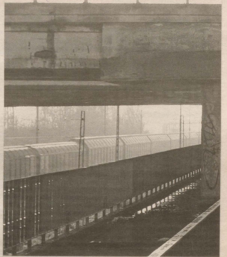
The term "wrong side of the tracks" came from the period when housing developments were built on one side of the city and industrial developments on the other side. / Stock photo
