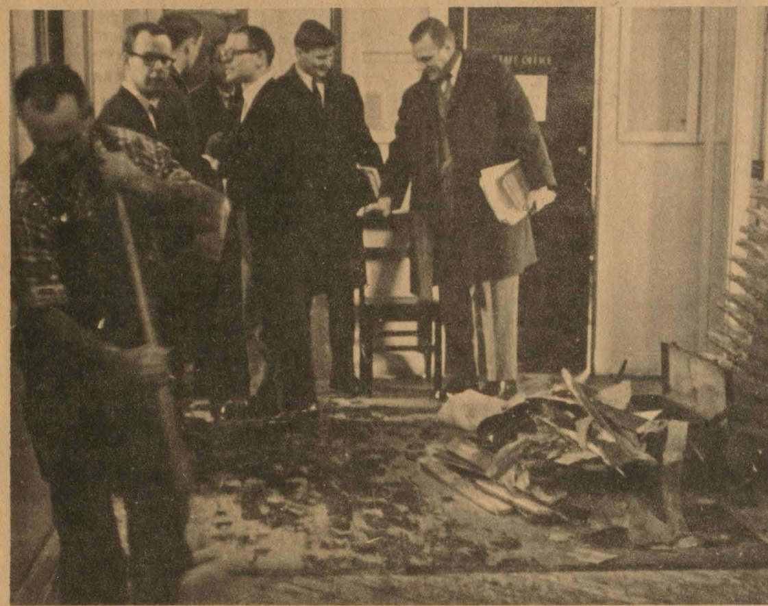
The workman is repairing the floor in the Arts Annex. Steam fittings broke below the wood timbers, causing them to swell and rise. Does this mark the beginning of the end for our beloved Arts Annex... only the Administration knows for sure.
