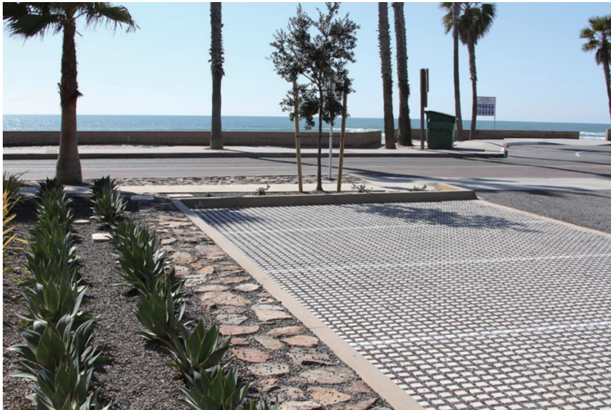
Drivable Grass® permeable pavers have many infill options including sand, rocks, ground cover, sod, stone, artificial turf and grass. Photograph by Jan Jansson, 2014
