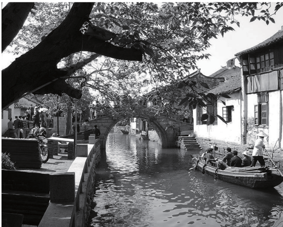
Open river side and footbridge
