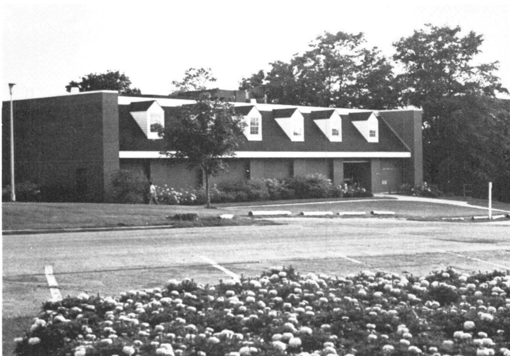
Jenkins Hall, NSAC's Dining Facility
