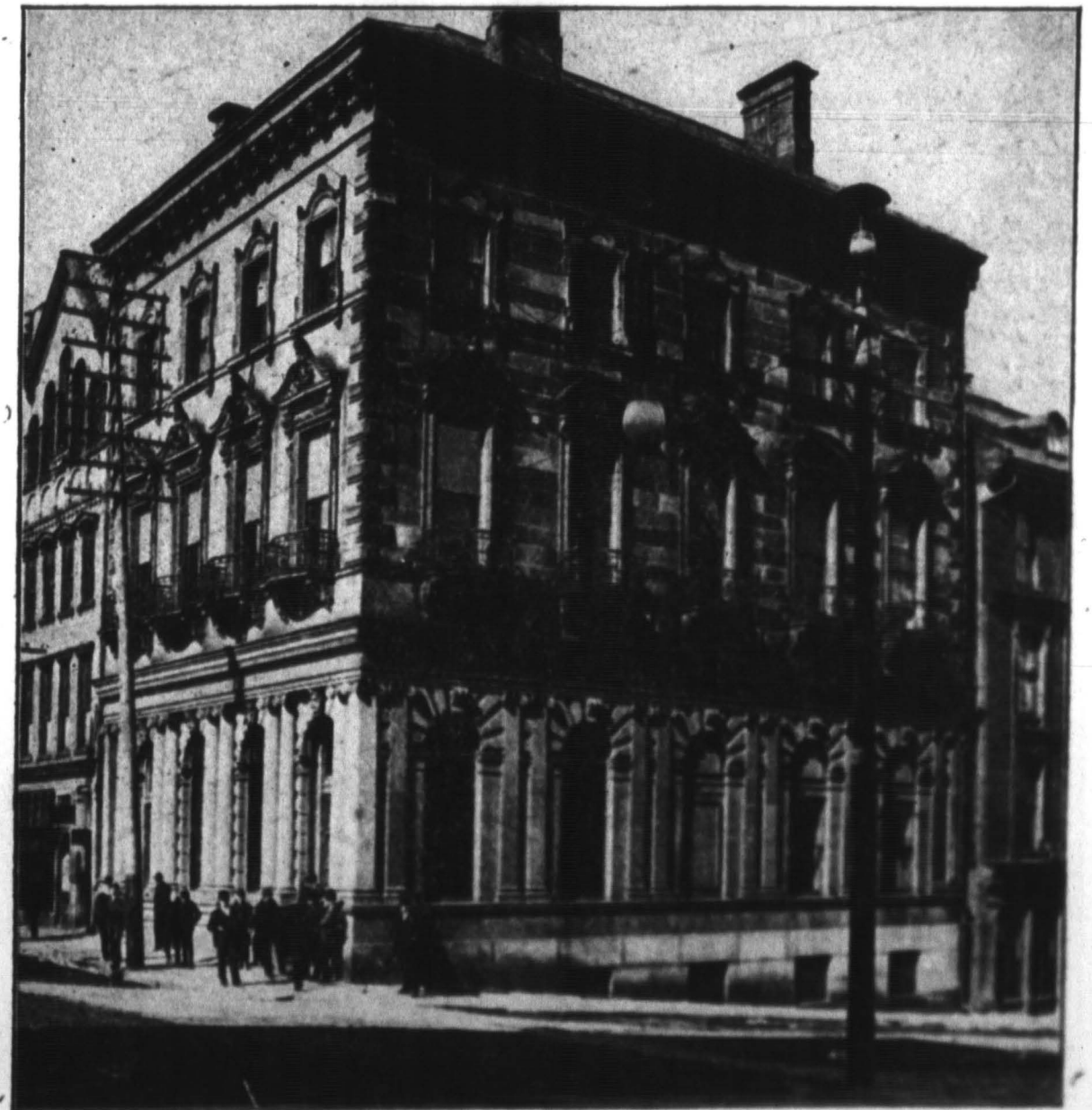
HOME OFFICE BUILDING
