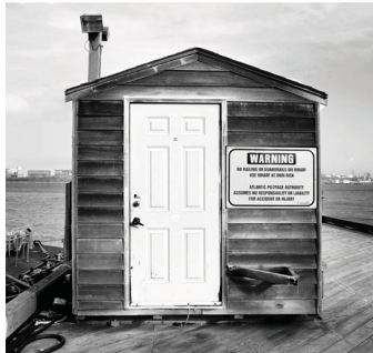
Small wharf shed building
