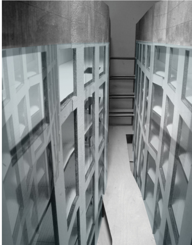
Continuous glazing over CLT structure of the central courtyard
