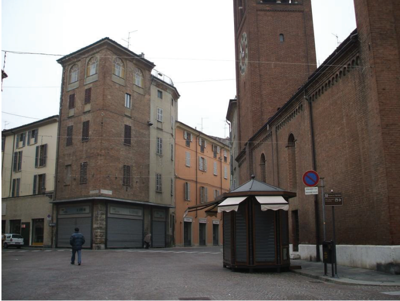
Figure 4-32: Piazza Borgo, with the church Santa Brigida to the right, fall 2010.
