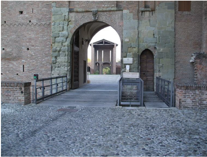
Figure 5-25: Entrance to main courtyard in Palazzo Farnese. December 2010.
