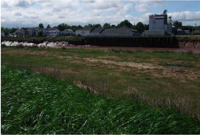
Figure 3.2 : Port William dyke protecting major road, residential, and commercial properties.
