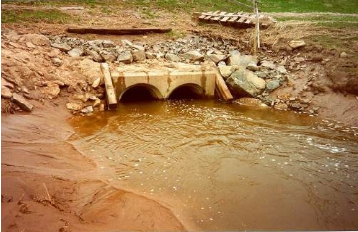
Figure 2.5: Modern materials (concrete) used in the construction of aboiteaux (Source: Nova Scotia Department of Agriculture, 2007)
