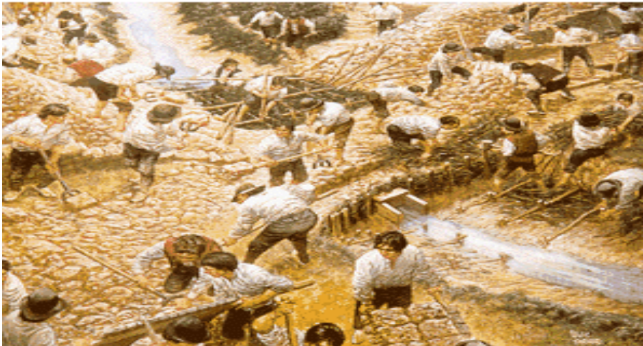
Figure 2.1: Dyke building in Acadia 1640-1650. The Acadians used simple tools to build and maintain the dykes and aboiteaux (Source: Consentino, 1998).
