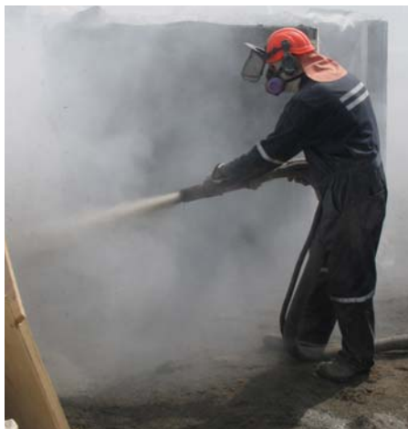
Figure 2.9 - Operation of a shotcrete hose
