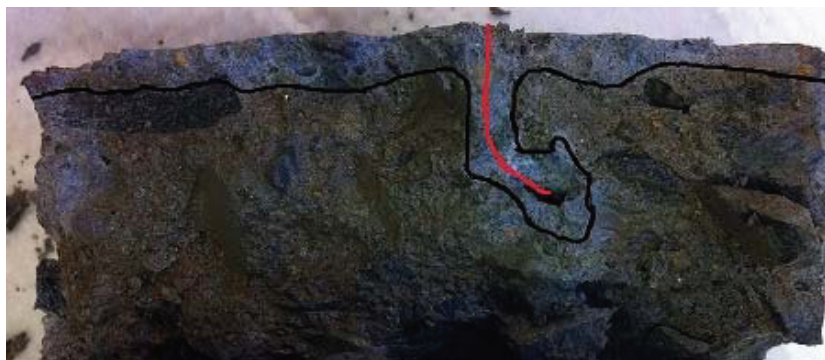
Figure 5.8 TER 50-1 Crack Close-up
