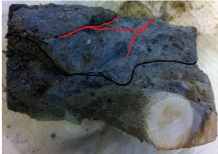
Figure 5.7 TER 50-2 Cracked Sample
