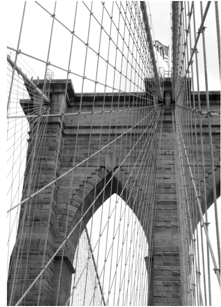
Brooklyn Bridge - suspension bridge.
