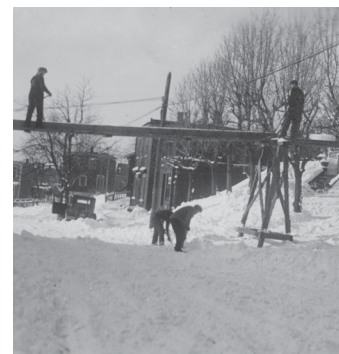
Ice being slid across Portland Street on a raised platform. From the Dartmouth Heritage Museum
