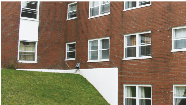
Existing unit entrance
