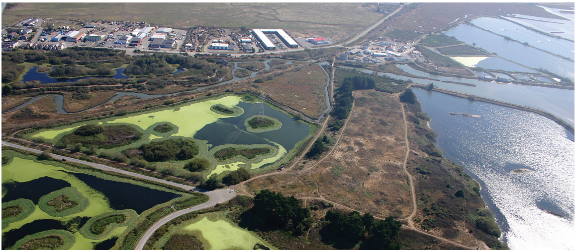
Aerial view of the marsh with wastewater treatment plant near the far upper right corner of image. (Arcata Marsh Overview 2008)
