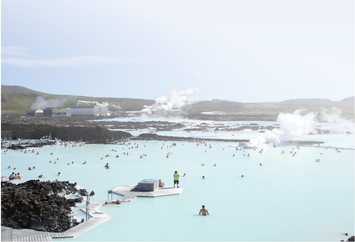
Svartsengi Power Plant and Blue Lagoon. From Terdiman, “Coder Corner.”
