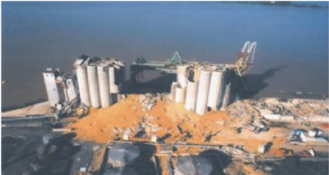
Figure 5.29 A view of the Semabla silo and warehouse-A storage facilities after the explosion (van der Voort et al., 2007).
