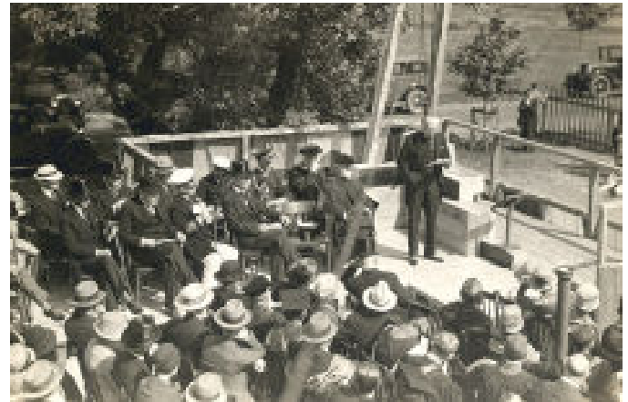
Nova Scotia premier Edgar N. Rhodes laying the cornerstone of the Chase Bldg., August 29, 1929 From: The Buildings of Dalhousie University
