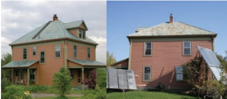
Solar power provides ~ 50% of the heat and electricity for Frank Fawson's century old farmhouse in Lunenburg County. Photo credit: Frank Fawson
