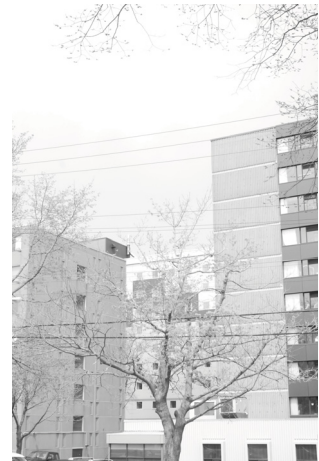
Looking from site across Northwood Terrace.
