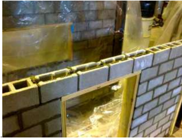
Figure 3.7 Bond beams and horizontal reinforcement
