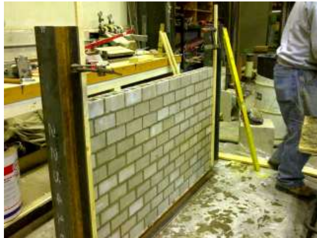
Figure 3.6 Pre-welded infill frames
