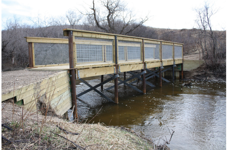
Creek valley bridge showing structure.
