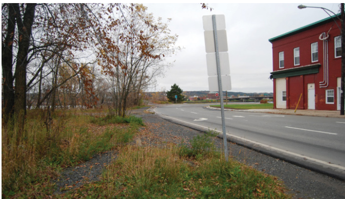
Dangerous curve as it approaches the unfinished walking trail.
