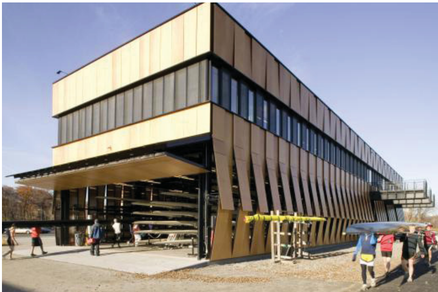
Harry Parker Boathouse with users storing boats. Pedestrian trail is shown in bottom right. Mechanical exterior walls can be seen allowing air circulation. (Image: Campbell, N.4.)
