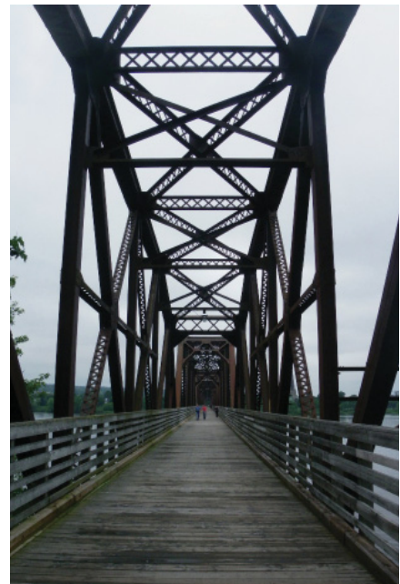
Wood deck of the Bill Thorpe Walking Bridge.
