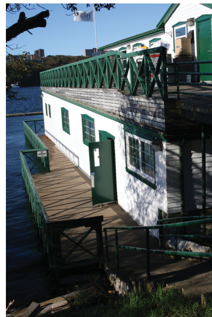
Side view of the St. Mary's Boat Club. Built almost entirely in the Northwest Arm, access to the reception hall ( top ) is by bridge, with the piers and storage accessed by stairs down the embankment.
