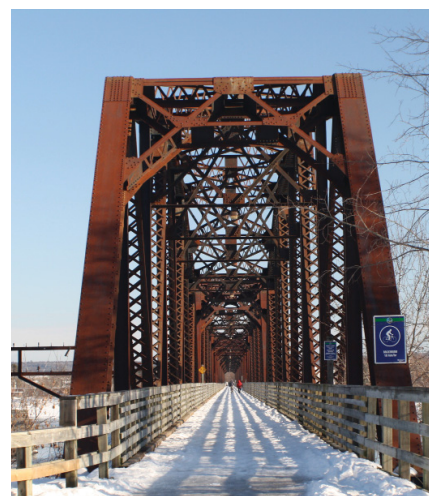
Bill Thorpe Walking Bridge, former train bridge converted for non-motorized recreation use in 1997. Spans 0.6km across Saint John River.
