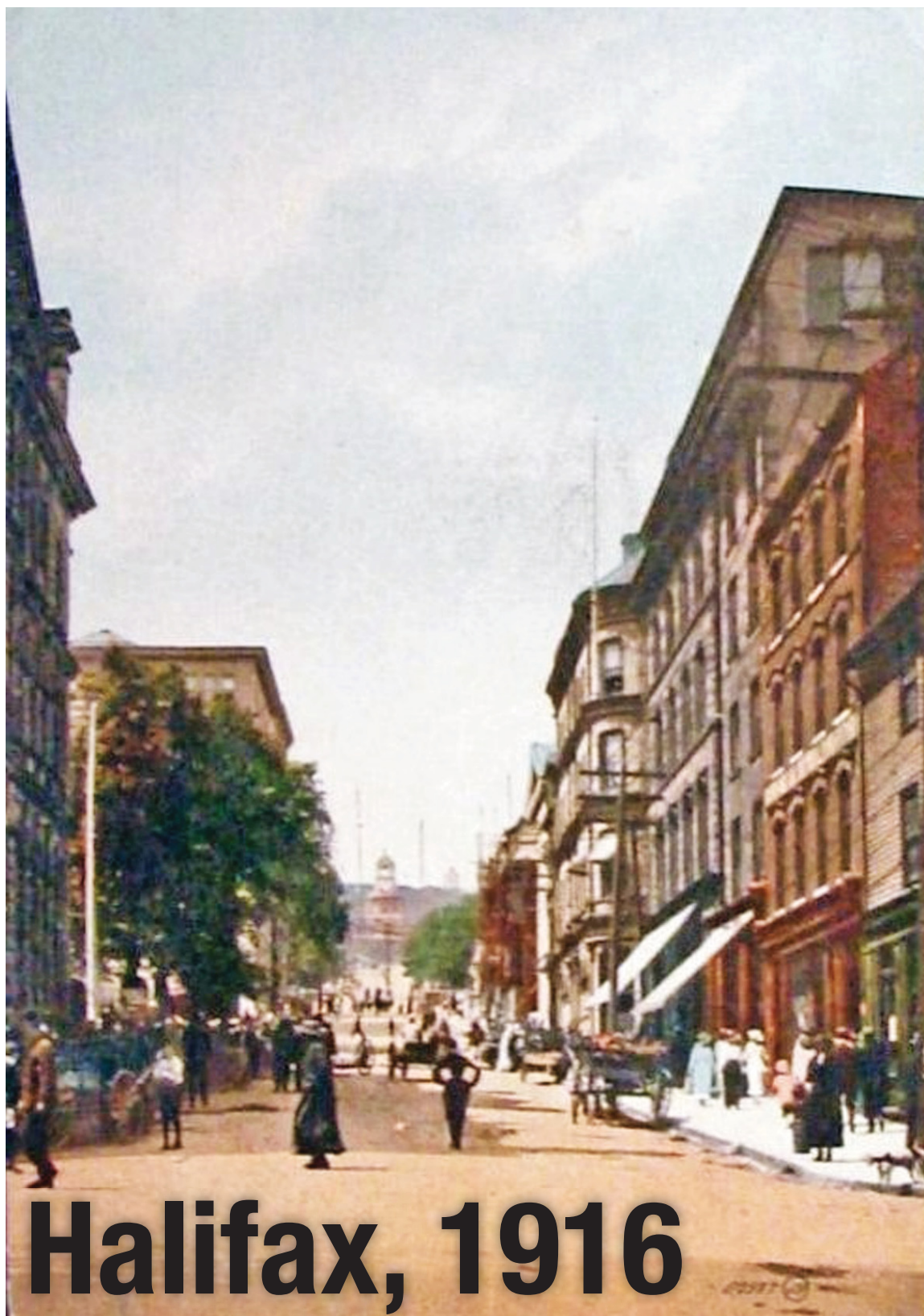
View looking up George Street towards the town clock, Halifax, Nova Scotia, 1916. Photographer Unknown. 'cooeypig', Flickr.
