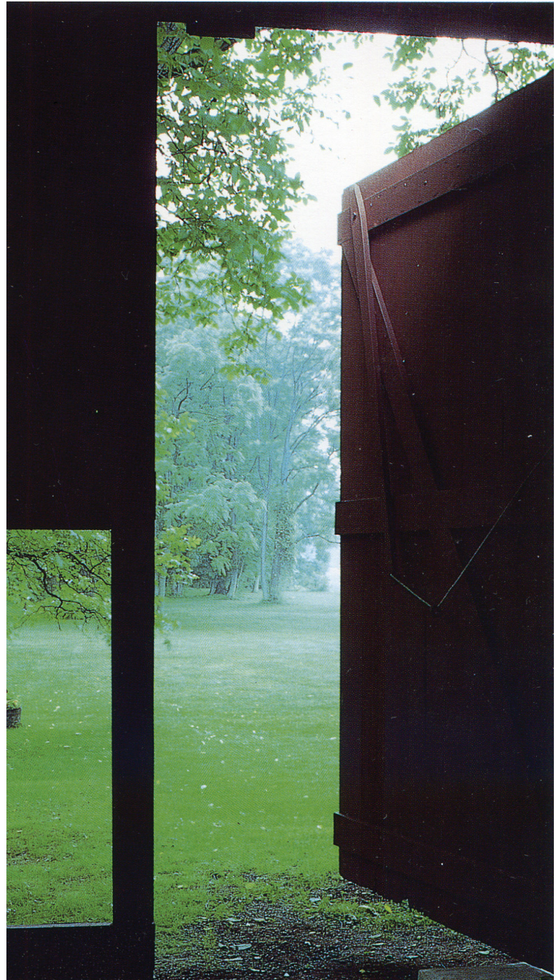
An alternative to previous image, Pennsylvania barn. Small door allows farmer daily access to barn without having to open larger barn door. Heat loss prevention in winter. Photograph by Paul Rocheleau, Barn: The Art of a Working Building .
