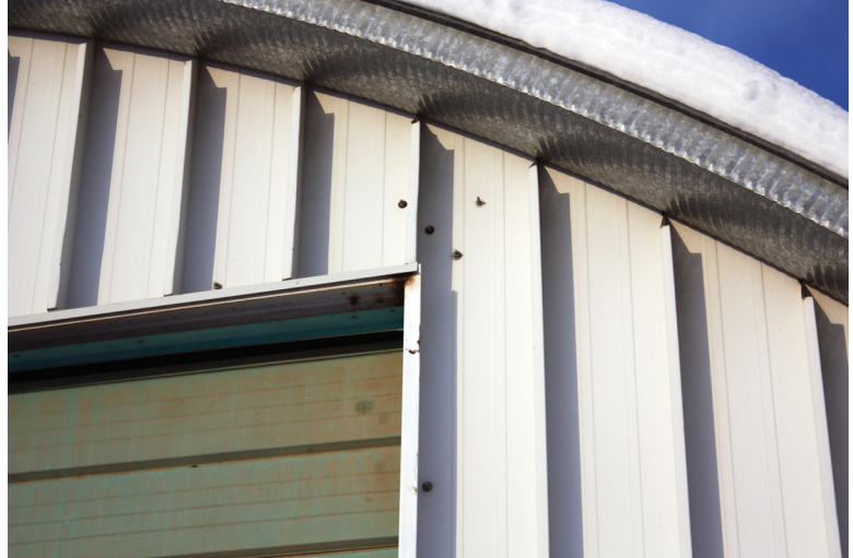
Machine shed 1 roof/eave detail, Manning, AB.
