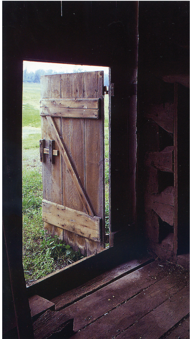
Large barn door to allow wagon access to threshing floor. A smaller access door within the large door helps to prevent heat loss from opening larger door during winter months while still allowing farmer daily access to the barn, Pennsylvania. Photograph by Paul Rocheleau, Barn: The Art of a Working Building .
