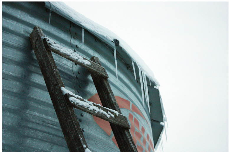
Round steel bin: built 1995, Manning, AB.
