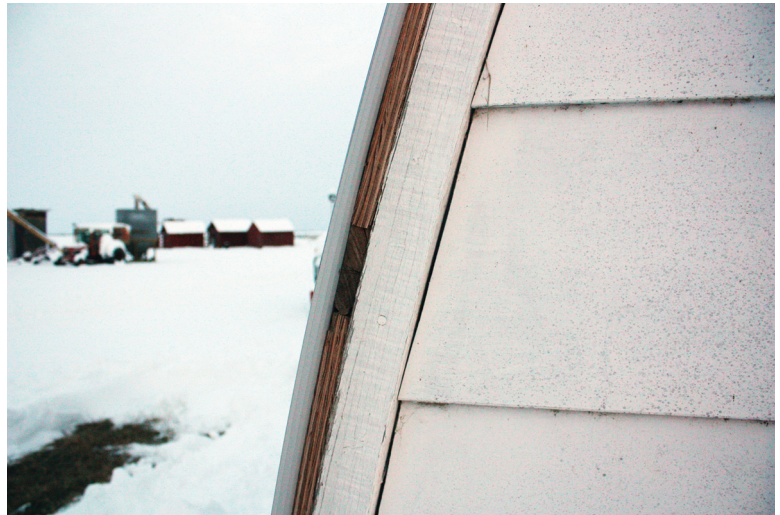
Machine shed 2 roof/eave detail, Manning, AB.
