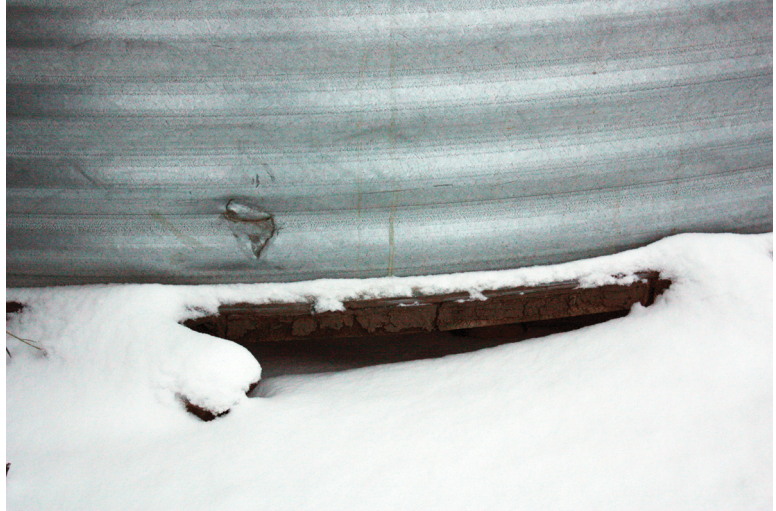
Steel bin to wood floor connection.
