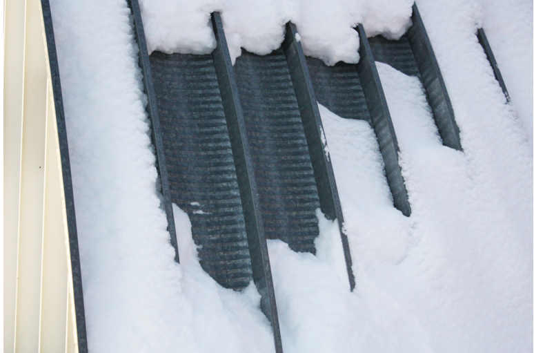
Machine shed: zip lock connection, Manning, AB.
