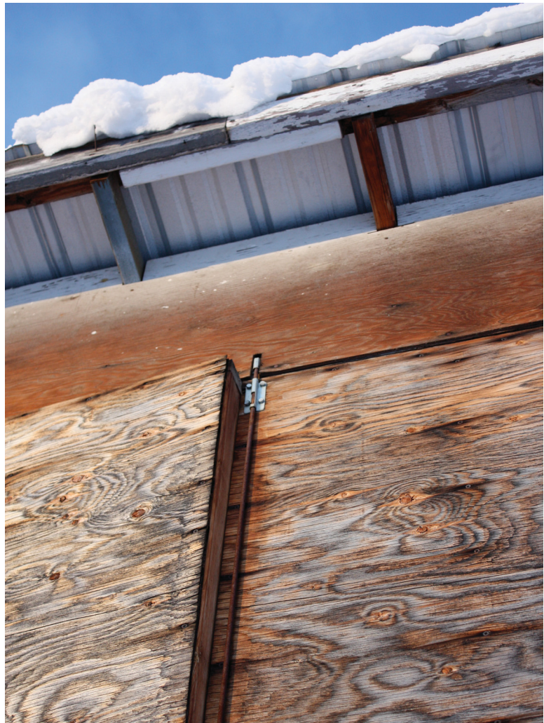
Seed cleaning shed door latch detail, Manning, AB.
