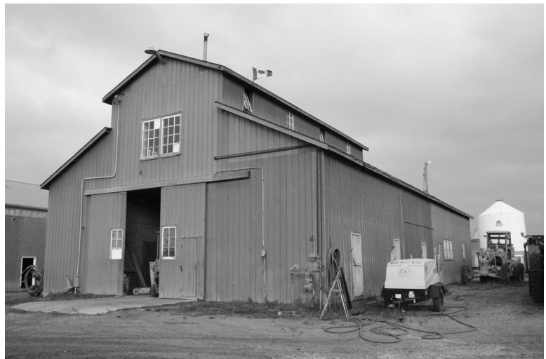
Seed cleaning shop: built 1962, Penhold, AB.
