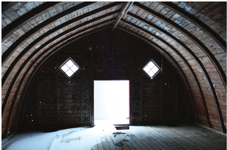
Barn loft interior structure, Manning, AB.
