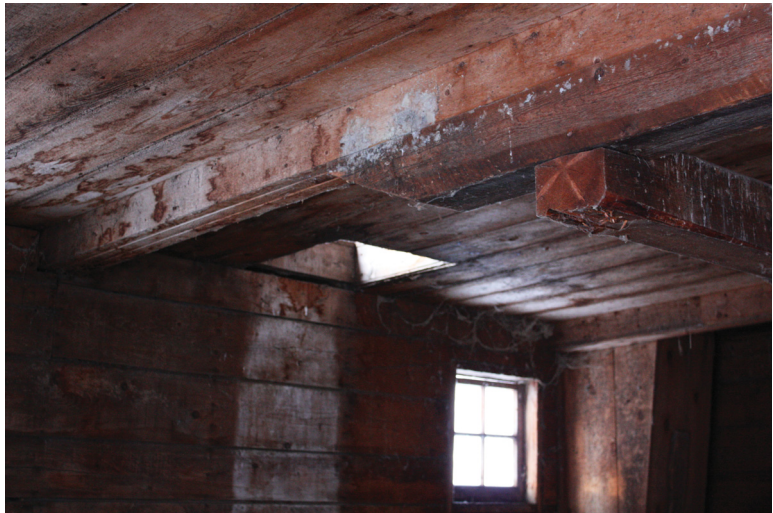
Barn interior: Cut-out in loft used for dropping whole straw bales to the level below. Straw is used for insulation as well as to layer over manure for odor management and animal/barn cleanliness, Manning, AB.
