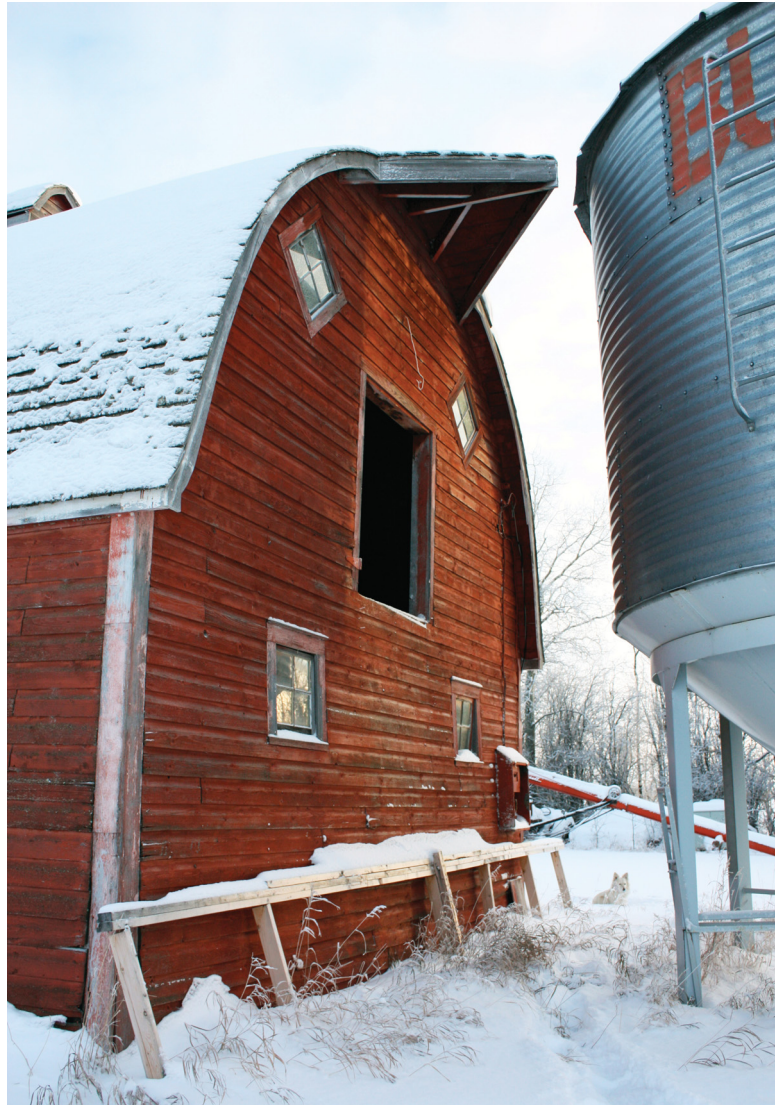
Barn: built 1940. Detail highlights extension of roof structure which held a large sling used to lift hay bails into loft prior to mechanical bale augers and bucket tractors. Steel hopper bin: built 2004, Manning, AB.
