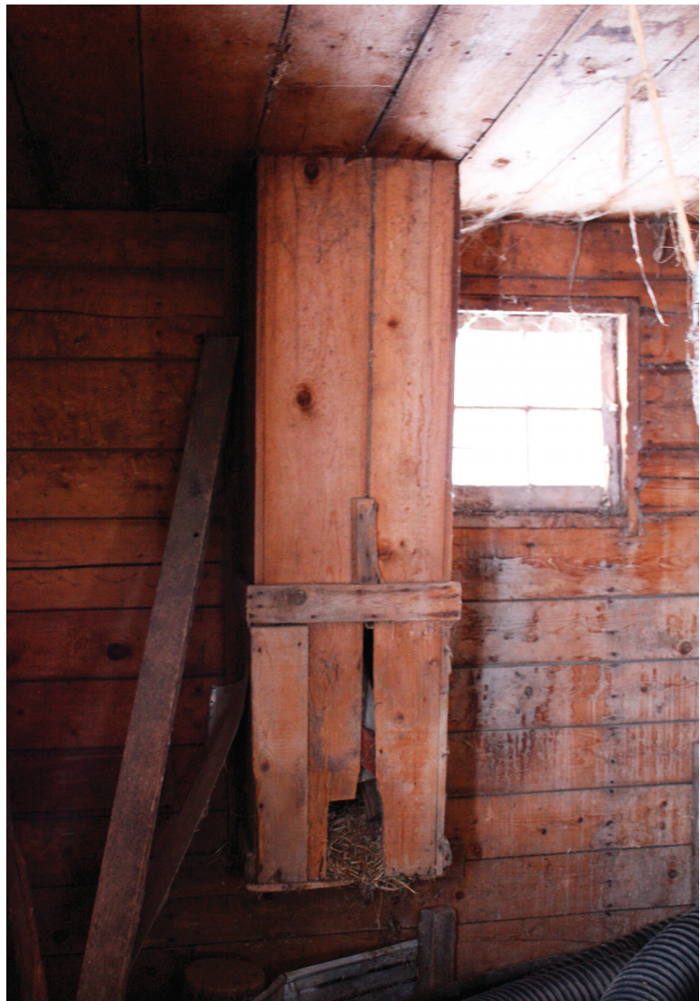
Barn interior: Hay chute from loft used to feed cattle during winter months, Manning, AB.
