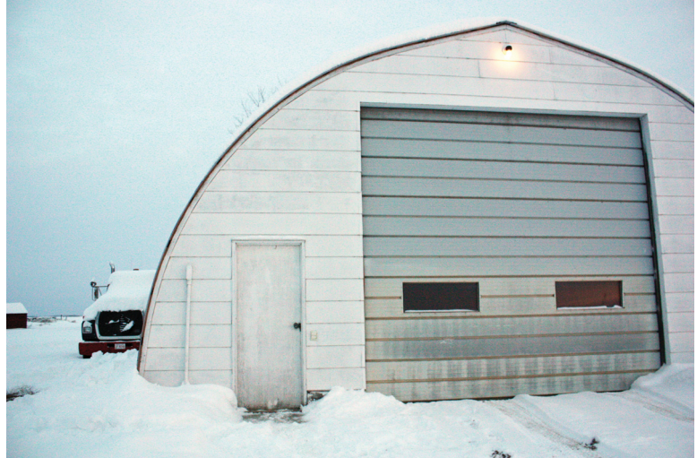
Machine Shop: built 1976, Manning, AB.
