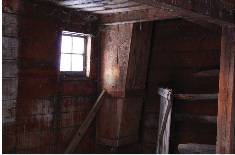
Barn interior: Hay chute [alternate view].
