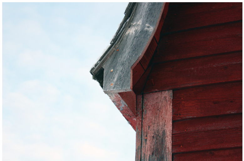
Barn eave detail: built 1940, Manning, AB
