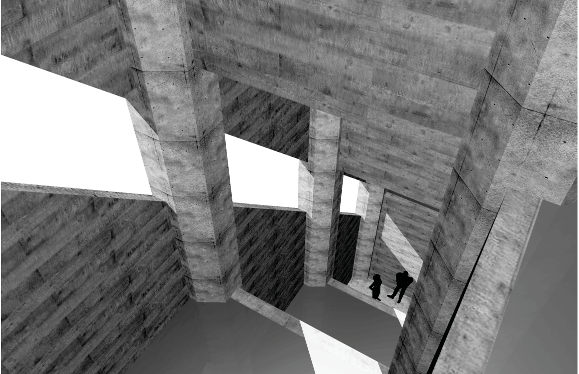
Figure 47: A series of rectangular openings are cut in the bin walls, floors are added at the base of the cut, and a diagonal slice is made in the exterior wall.
