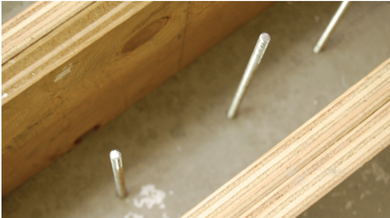
The threaded rod supports were hammered into the predrilled holes.
