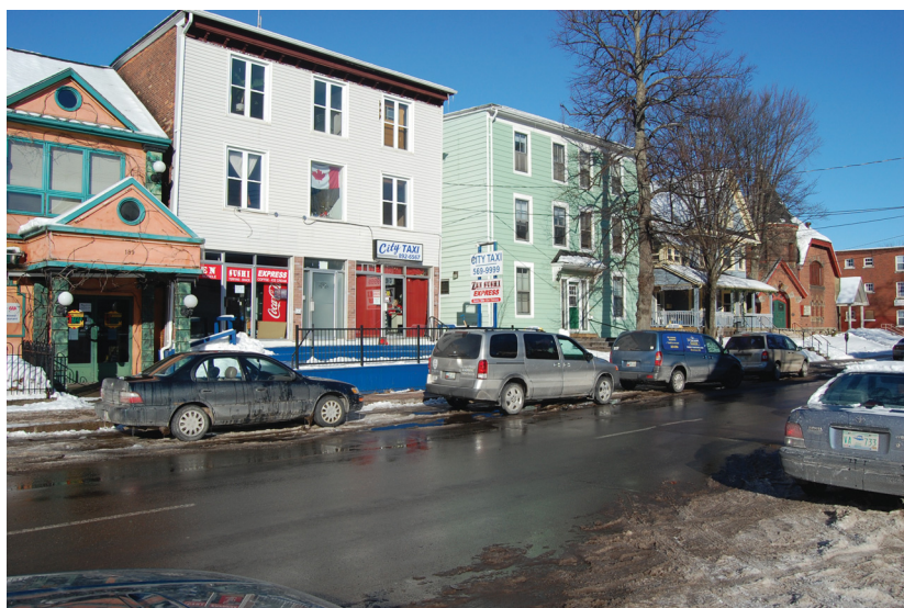
(Top) Central Christian Church, Kent Street, Charlottetown, Prince Edward Island. (Bottom) Mixed Use Buildings, Kent Street, Charlottetown, Prince Edward Island.
