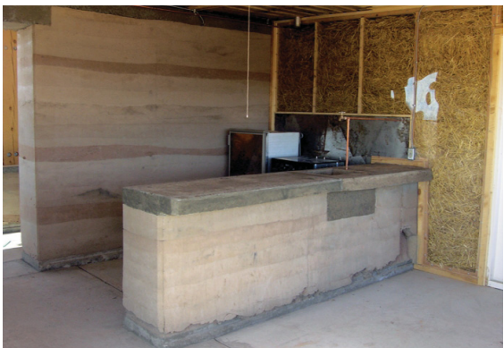
Rammed Earth Trombe Wall, Interior and Exterior Views, Rosie Joe House, Teec Nos Pos. Photographs from "Design Build Bluff: Sustainable Homes For People Who Need Them."
