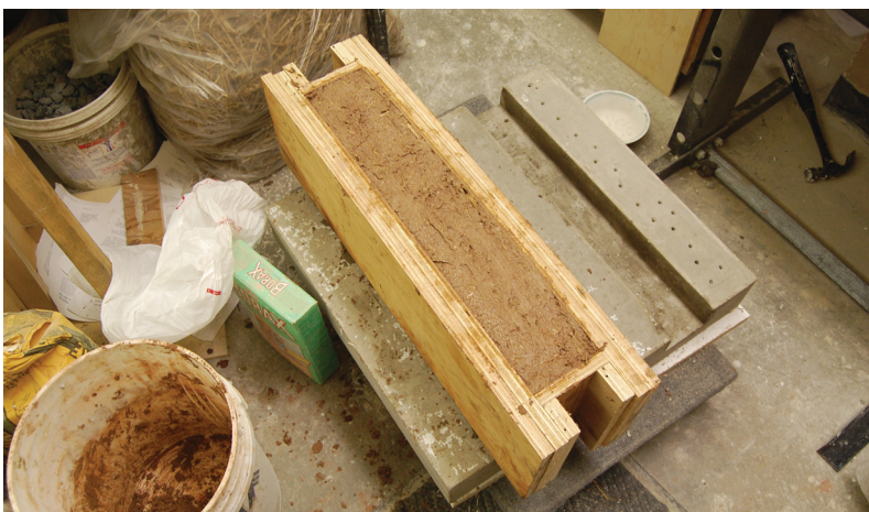
The rammed earth section is completed and left to dry.
