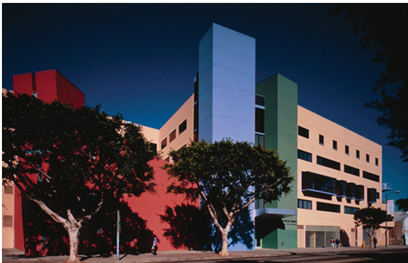
Front Facade, Union Rescue Mission, Los Angeles. Photograph from Designing for the Homeless: Architecture that Works .
