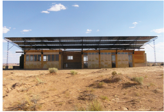
Rammed Earth Trombe Wall, Interior and Exterior Views, Rosie Joe House, Teec Nos Pos. Photographs from "Design Build Bluff: Sustainable Homes For People Who Need Them."
